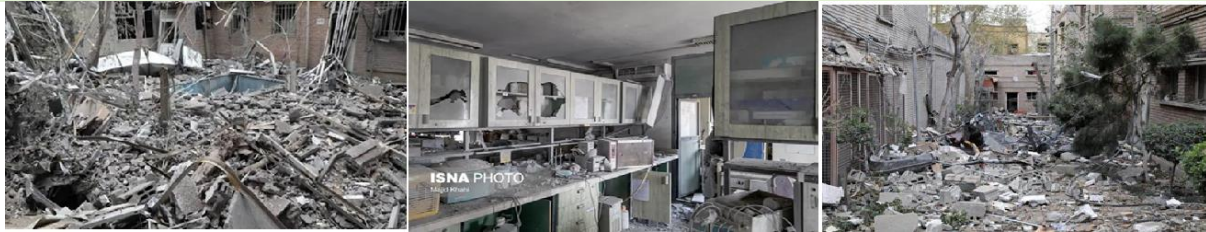
Figure 9. Damage to the Pasteur Institute of Iran Following the Reported Strike, Including Structural Damage and Impacts on Research and Laboratory Facilities. Sources: Iranian Students' News Agency (ISNA) and Tabnak, (2026).
